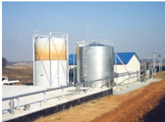
Figure 6. Biogas plant digesting pig manure of 10 m 3 /d at Seung Hwan, Korea.
