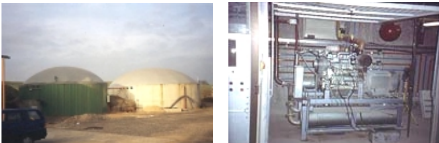
Figure 5. BARZ cofermentation biogas plant and co-generator, Germany.
