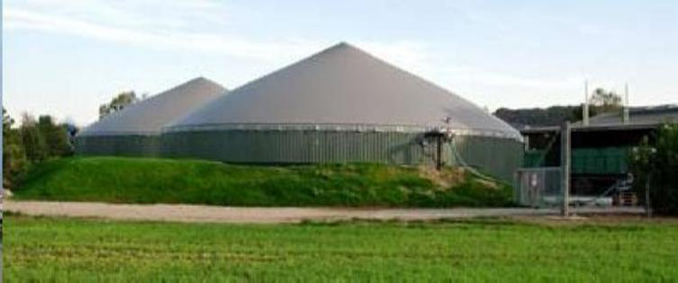
**Flat digester with gas holder roof**
