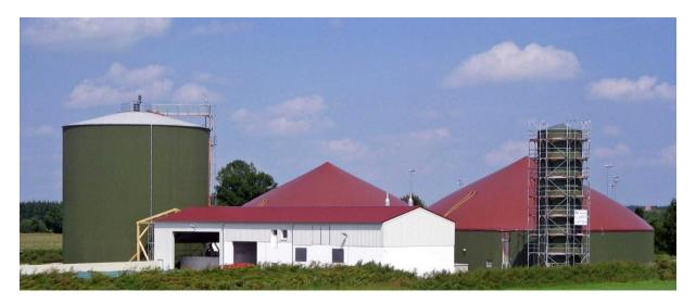
Location: Construction Period: Input: Fermenter: Co-generator: Special Features: Buchloe, Bavaria, Germany 2006 Maissilage, GPS, Grassilage Glass coated steel tank, 4.610 m<sup>3</sup>  $2 \times 526 \text{ kW}_{el}$  gas engines Gas holder above storage tank, pure energy crop digestion without addition of manure, thermophilic operation, full heat recovery
