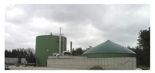
Location:GermanyConstruction Period:2005Input:Cattle Manure and Dung, Grass and Corn SilageFermenter:Concrete Tank, 2,616 m³Co-Generator:Gas engine, 526 kWSpecial Features:Double Membrane Gas Holder Roof, Separate Building<br/>for all Equipment incl. CHPCosts:about € 1,500,000.-
