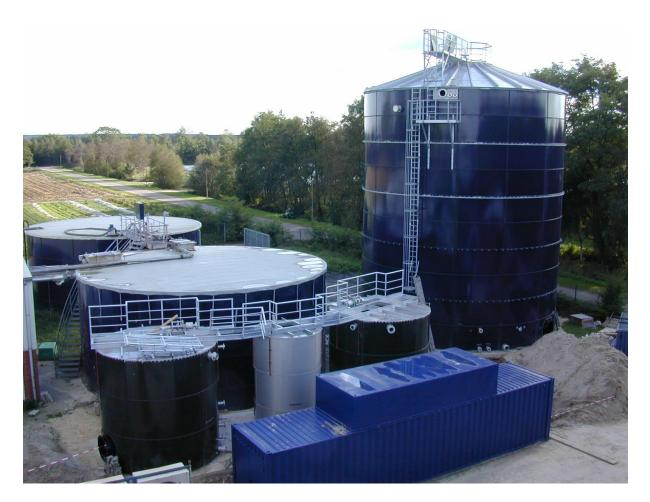
Location: Construction Period: Input: Fermenter: Co-generator: General Contractor: Germany 2002/2003 Manure, Fats Steel Tanks, 2 x 500 m<sup>3</sup> (original), 1,500 m<sup>3</sup> (additional) Gas Engines, 285 kW (original), 626 kW (additional) Hese Umwelt GmbH
