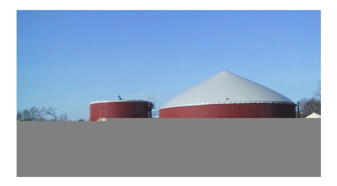
Location: Construction Period: Input: Fermenter: Co-generator: Costs: Germany 2002/2003 Manure, Vegetable Fats and Oils Concrete tank, 445 m<sup>3</sup> Gas Engines, 100 kW, 70 kW æì∫ čớk ÁH € €€€€
