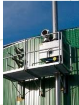
Overpressure- vacuum relief valve
