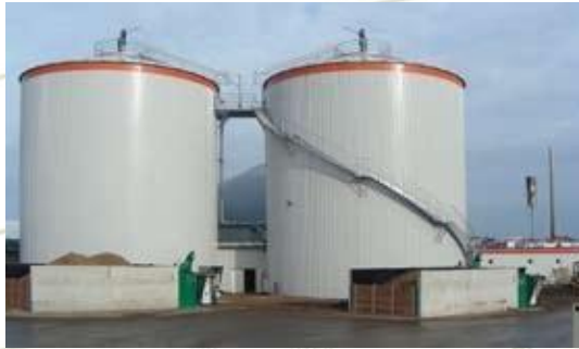
High upright digester
