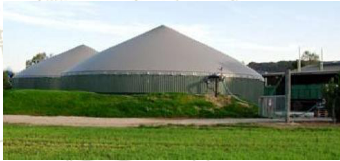
Flat digester with gasholder roof
