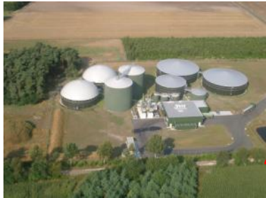
Central Biogas Plant
