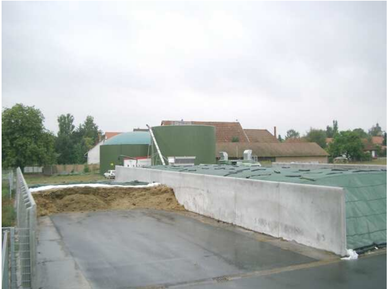
Fig. 1: Biological gas facility OBERNJESA
