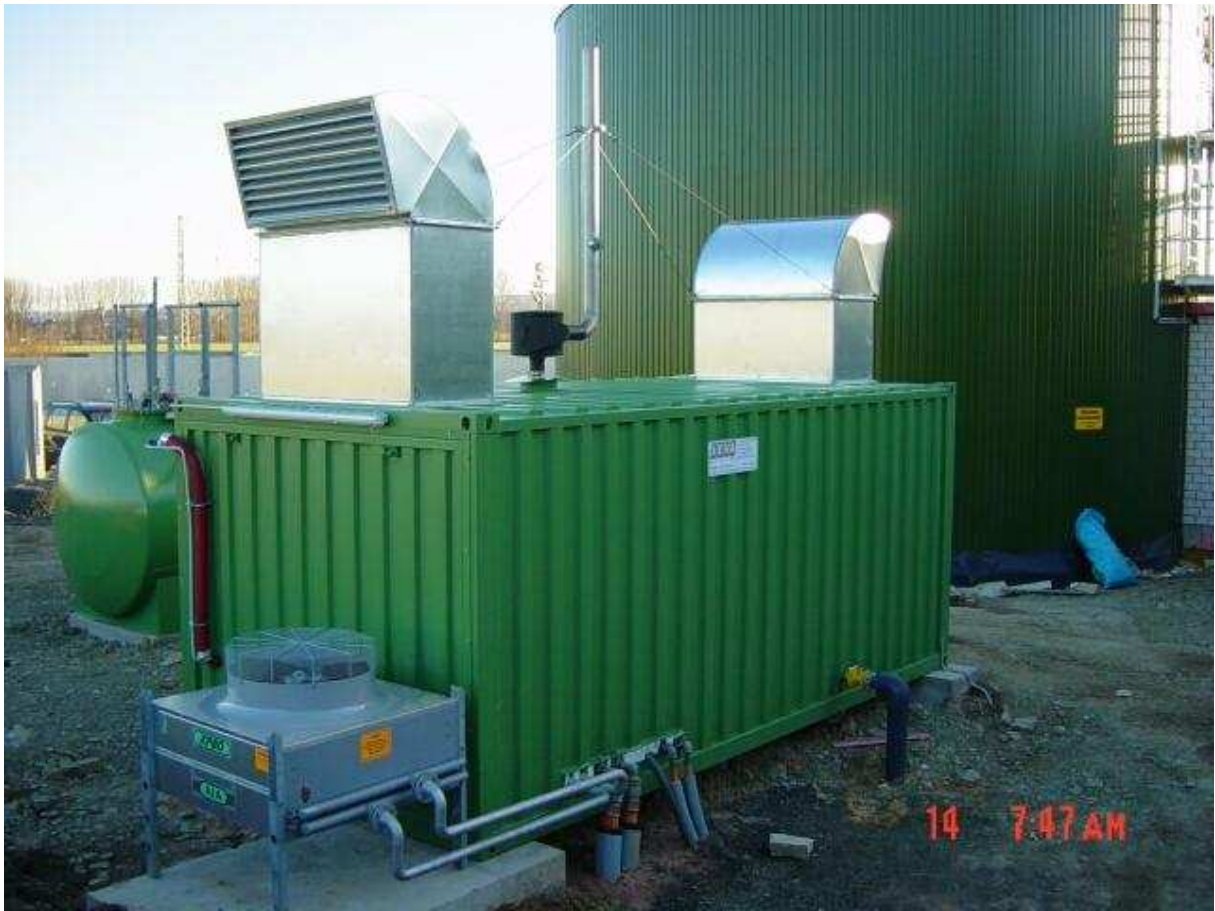
Fig. 4: (Combined Heat and Power (CHP) Plant alongside the fermenter. Biogas-Blockheizkraftwerk = BHKW)
