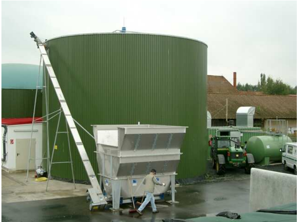
Fig. 3: Primary fermenter, solid input device in the foreground. Notice the inflated gasholder roof on the secondary digester behind the left side of the primary digester and the dual fuel CHP to the right.
