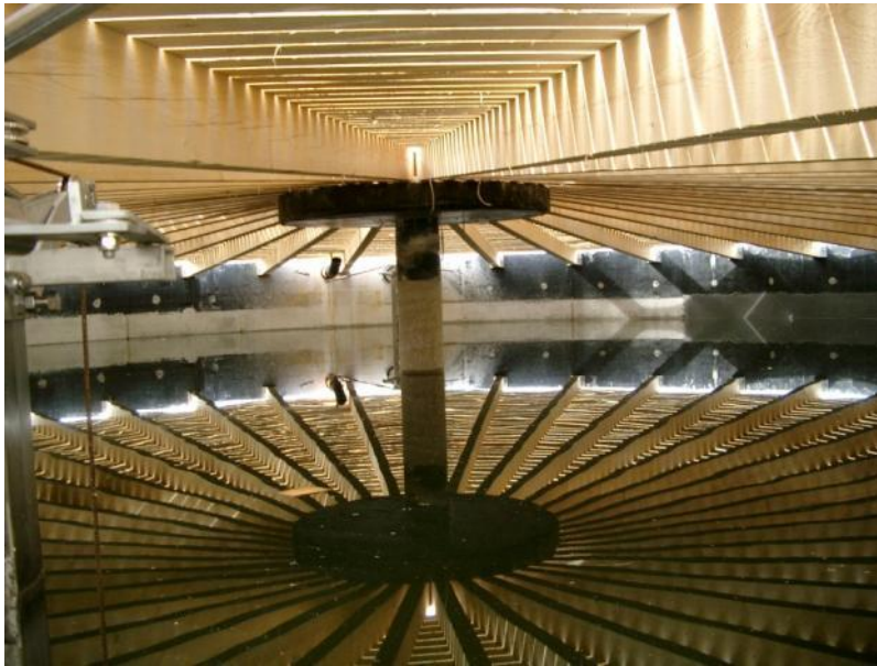
Wood construction in the secondary digester tank
