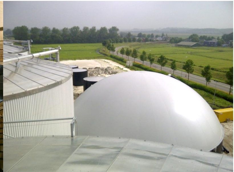
Gas holder on top of secondary digester tank
