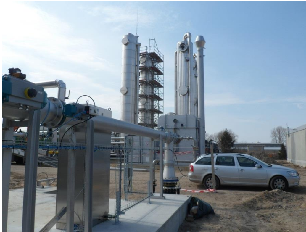
Biogas upgrading and injection of bio-methane into the natural gas grid
