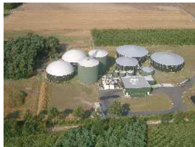
Central Biogas Plant
