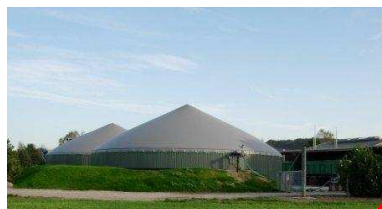
Kitchen Waste Digestion
