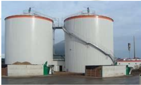
High upright digester
