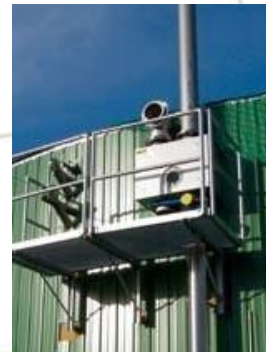
Overpressure- vacuum relief valve
