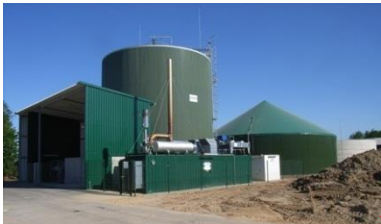
Energy Crop Biogas Plant
