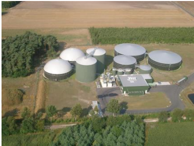
Central Biogas Plant
