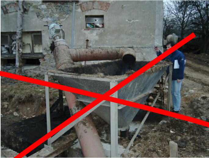
Food waste injection point
