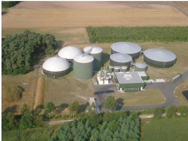
Central Biogas Plant
