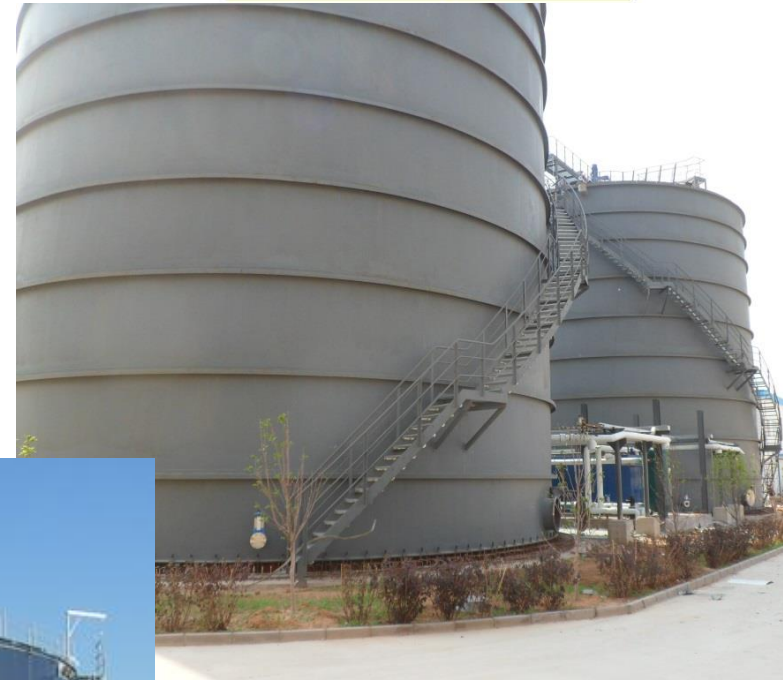
Welded steel tanks China
