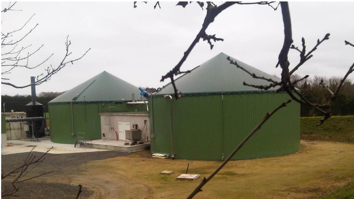
Secondary Digester B401 1.060 m 3
