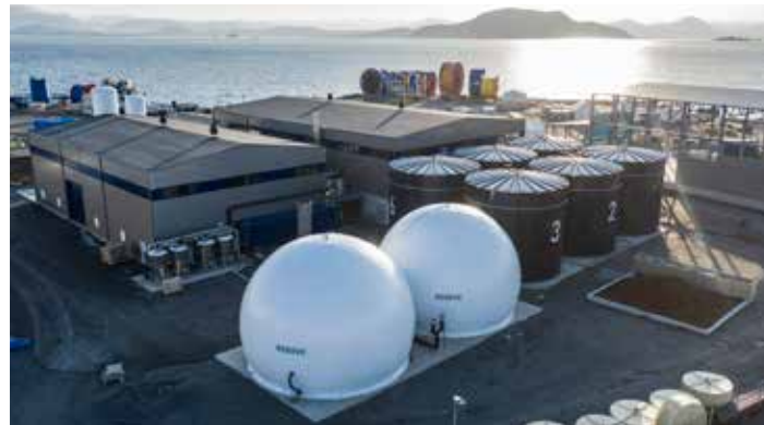
RENEVO's Renewable Energy plant in Stord. Photo credit: RENEVO
